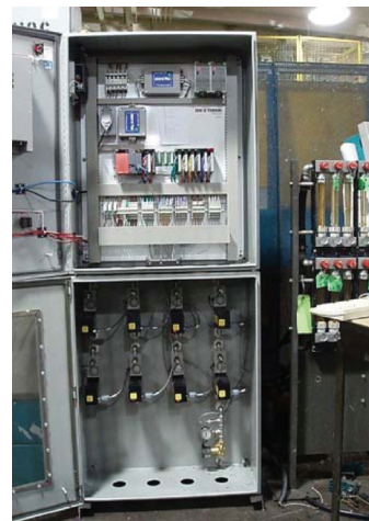
Figure 5 – Photograph of a DTE cooling line water control system.
